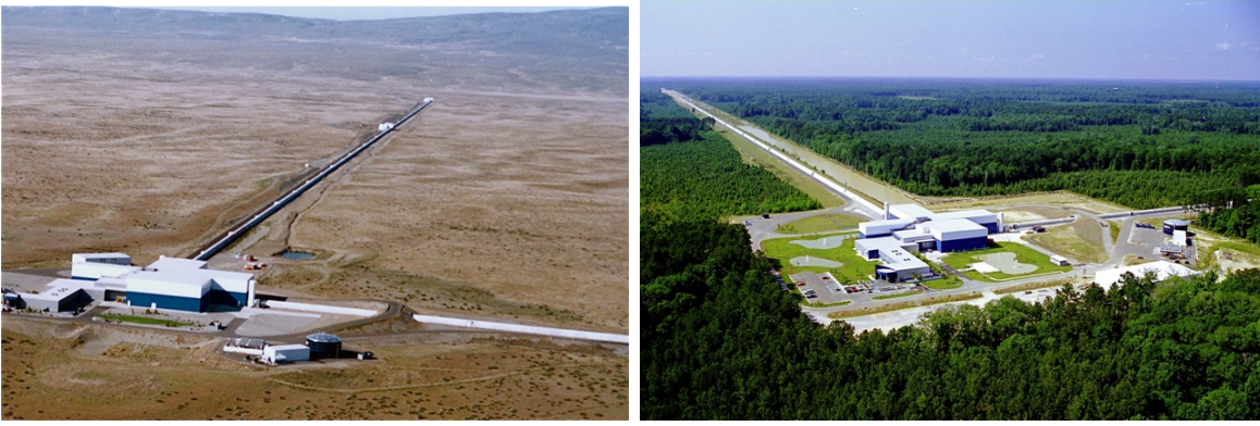
Figure 8: Aerial photographs of the LIGO observatories at Hanford, Washington (left) and Livingston, Louisiana (right) [94]. The lasers and optics are contained in the white and blue buildings. From the large corner building, evacuated beam tubes extend at right angles for 4 km in each direction (the full length of only one of the arms is seen in each photo); the tubes are covered by the arched, concrete enclosures seen here. Credit: LIGO Laboratory.
