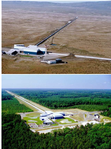
Figure 1.1 Aerial photograph of the LIGO observatories at Hanford, Washington (top) and Livingston, Louisiana (bottom). The lasers and optics are contained in the white and blue buildings. From the large corner building, evacuated beam tubes extend at right angles for 4 km in each direction (the full length of only one of the arms is seen in each photo); the tubes are covered by the arched, concrete enclosures seen here.
